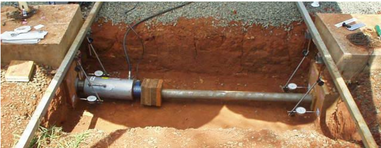
Figure 3: View of the Load Test Assembly
