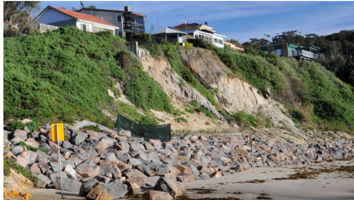
Figure 1. Rock-armoured revetment, Cabbage Tree Harbour, NSW, Australia (photo: A Nielsen)
