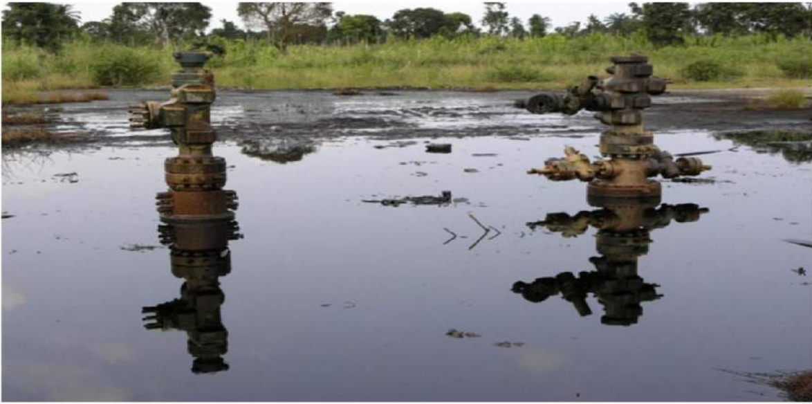
Picture Showing a Leaked oil well at Elume Village
