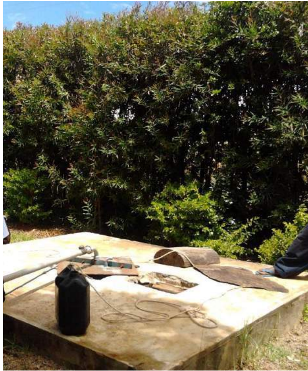
Figure 4: Protected well within a medium farm size showing modes of water extraction using a bucket and rope
