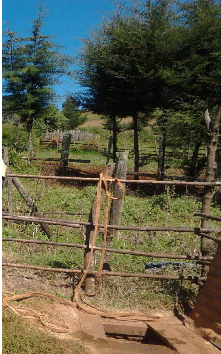
Figure 3: Close up of the semi-protected well in Fig. 2
