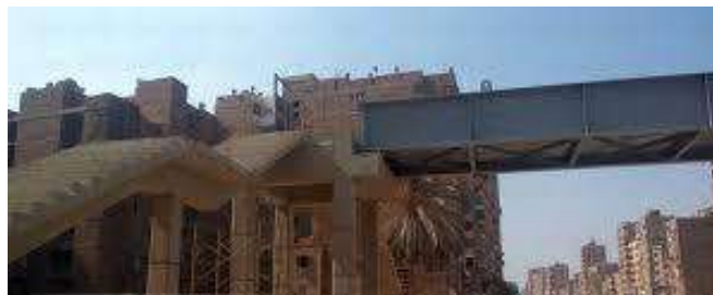
Fig. 1: Photo of Stair
