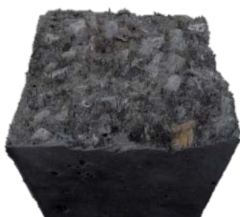
Figure 5: Appearance of the Fibers on the Casting Concrete Surface
