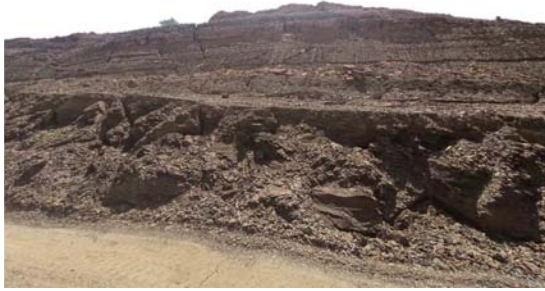
(a) Jinyang highway landslide
