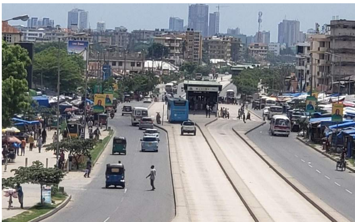
Figure 2: Manzese BRT bus stop Dar es Salaam City
