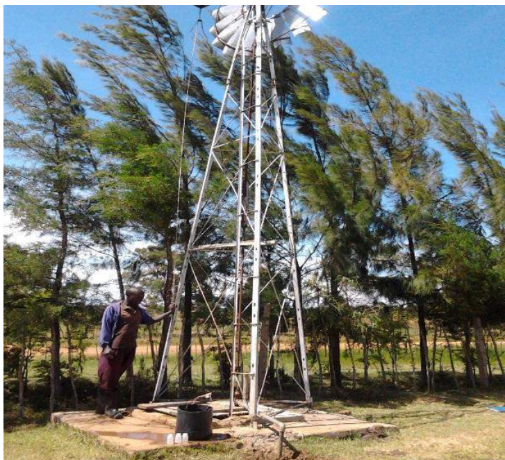
Figure 5: Protected wells within the medium farm sizes showing windmill mode of water extraction
