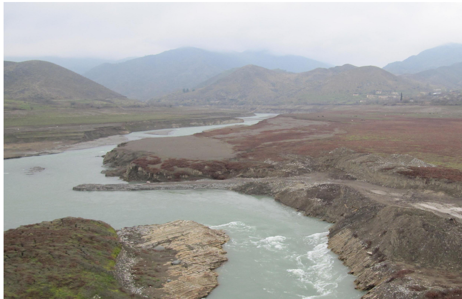
Fig. 6: Flushing ravine in the sediments of the Mataghis reservoir
